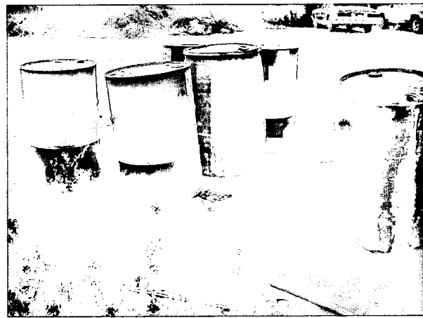
Photo 10: Above ground diesel tank with discharge onto soil.
