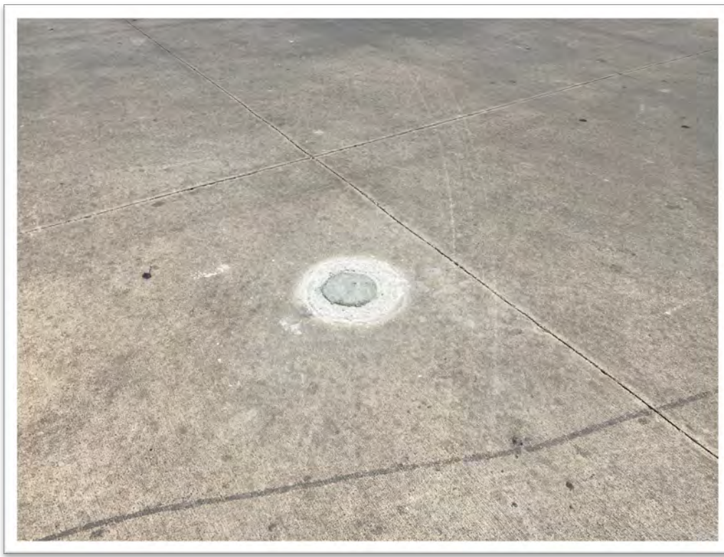
PHOTOGRAPH 5 – VIEW OF MW-4 POST WELL PLUGGING WITH CEMENT
