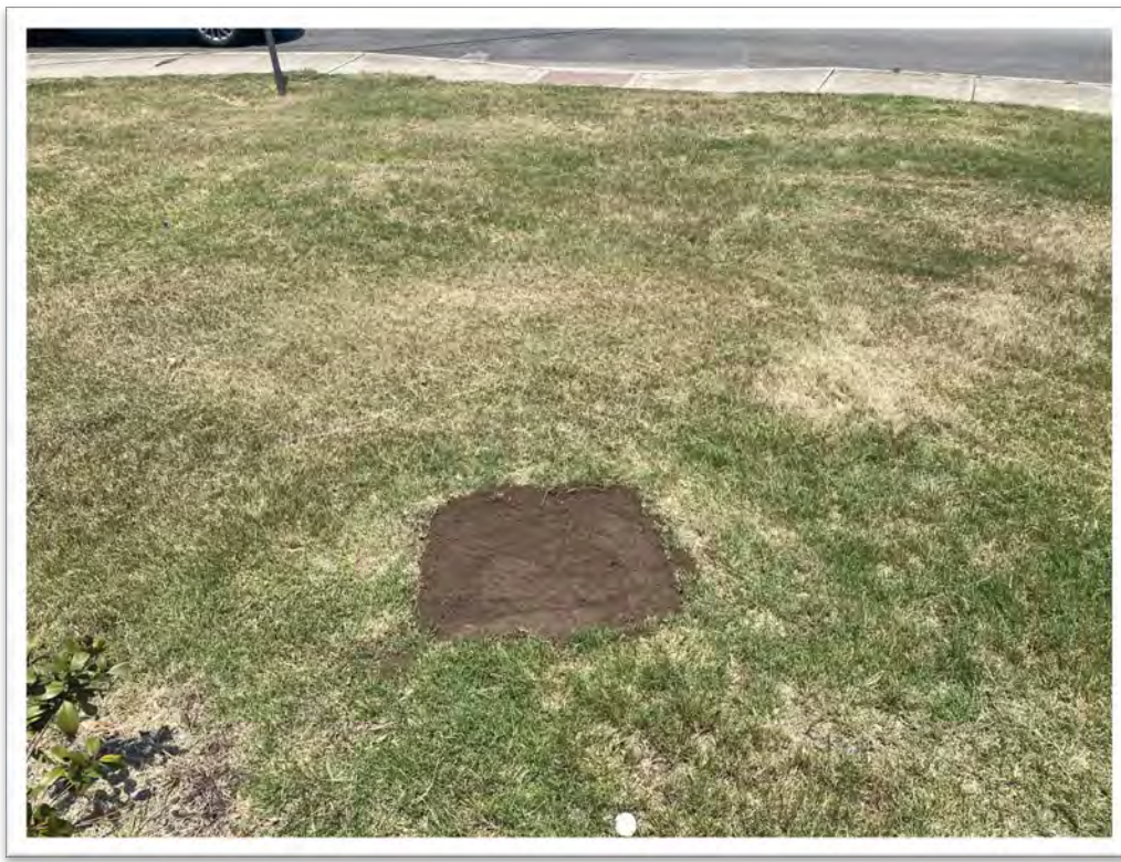
PHOTOGRAPH 9 – VIEW OF MW-5 POST WELL PLUGGING WITH TOPSOIL
