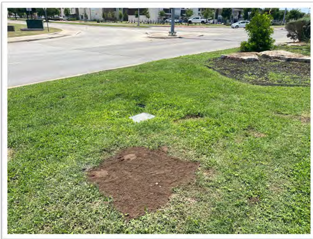
PHOTOGRAPH 7 – VIEW OF MW-8 POST WELL PLUGGING WITH TOPSOIL
