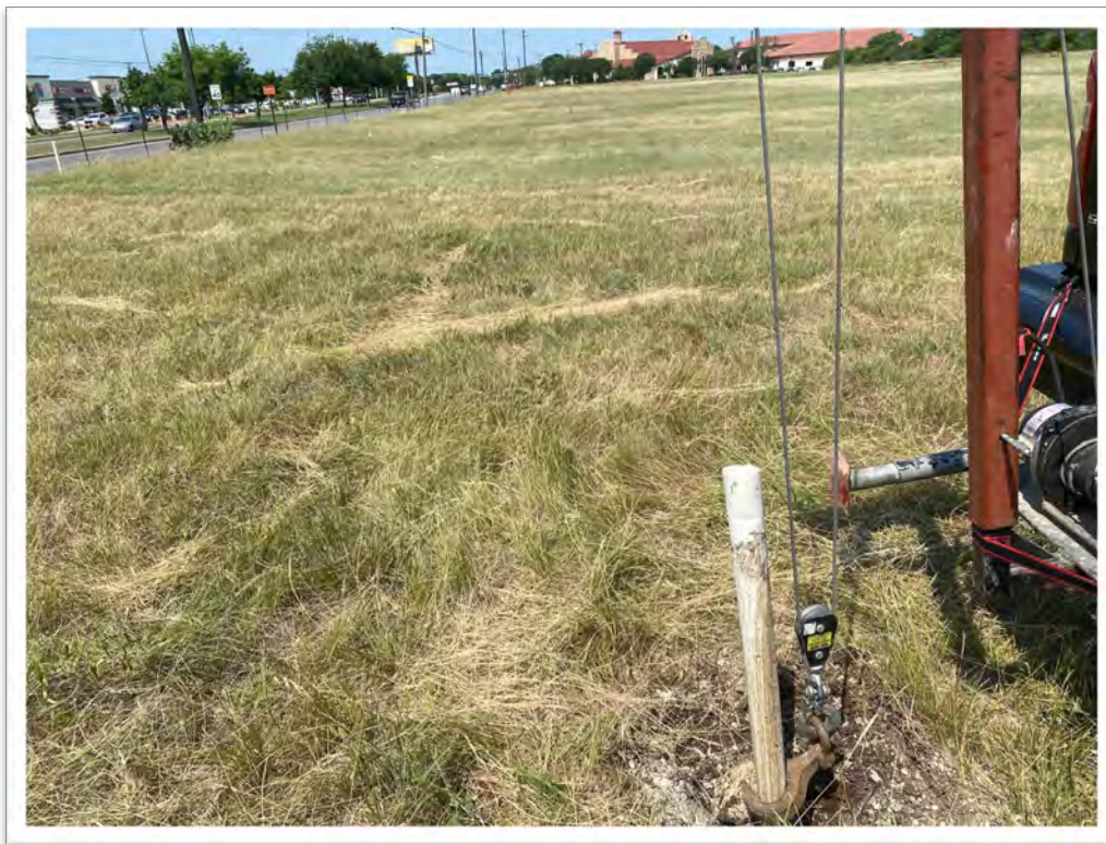
PHOTOGRAPH 3 – VIEW OF PULLING WELL CASING ON MW-9
