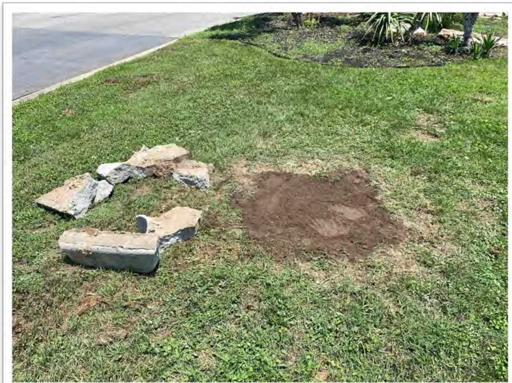
PHOTOGRAPH 6 – VIEW OF MW-7 POST WELL PLUGGING WITH TOPSOIL. THE WELL PAD MATERIALS WAS SUBSEQUENTLY REMOVED FOR DISPOSAL.
