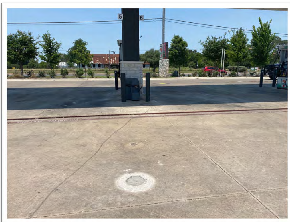
PHOTOGRAPH 8 – VIEW OF MW-3 POST WELL PLUGGING WITH CEMENT
