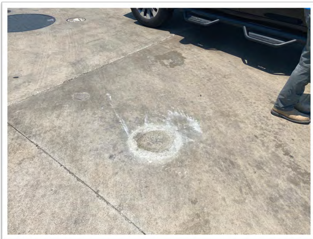
PHOTOGRAPH 10 – VIEW OF MW-1 POST WELL PLUGGING WITH CEMENT
