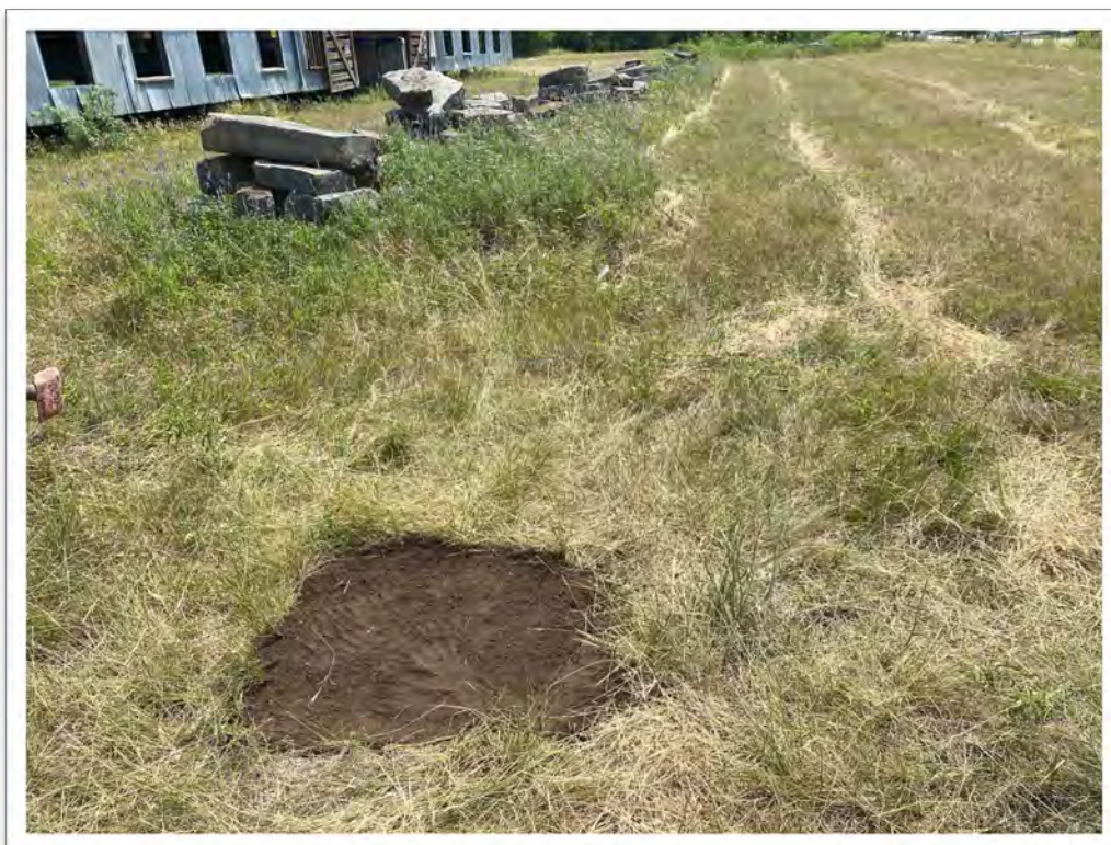
PHOTOGRAPH 4 – VIEW OF MW-9 POST WELL PLUGGING WITH TOPSOIL
