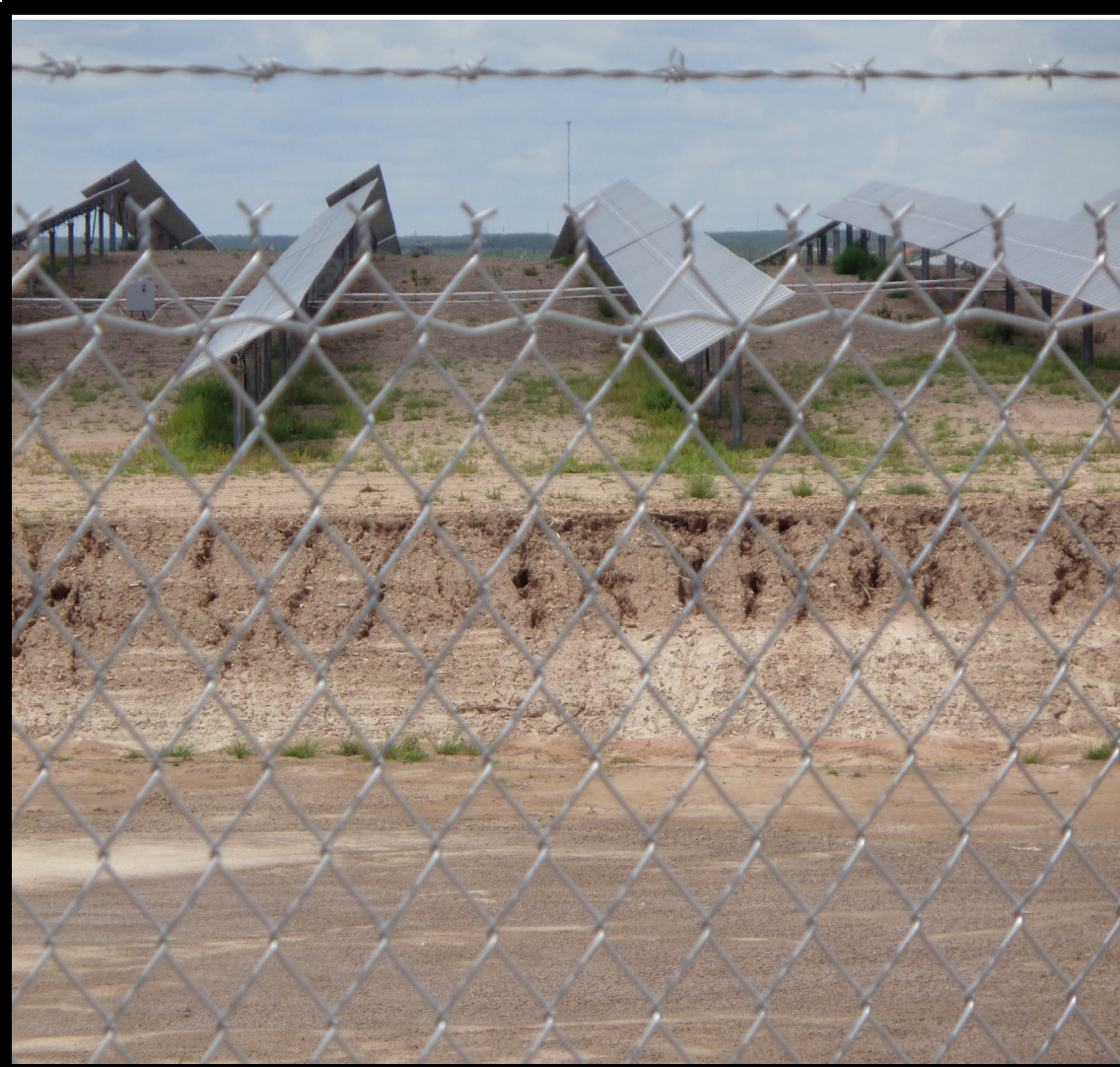
Eroded wall at detention pond
